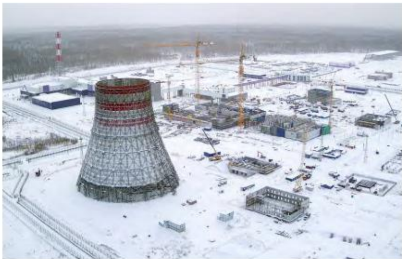
Pilot Demonstrational Energy Complex (PDEC), in construction © SCC
